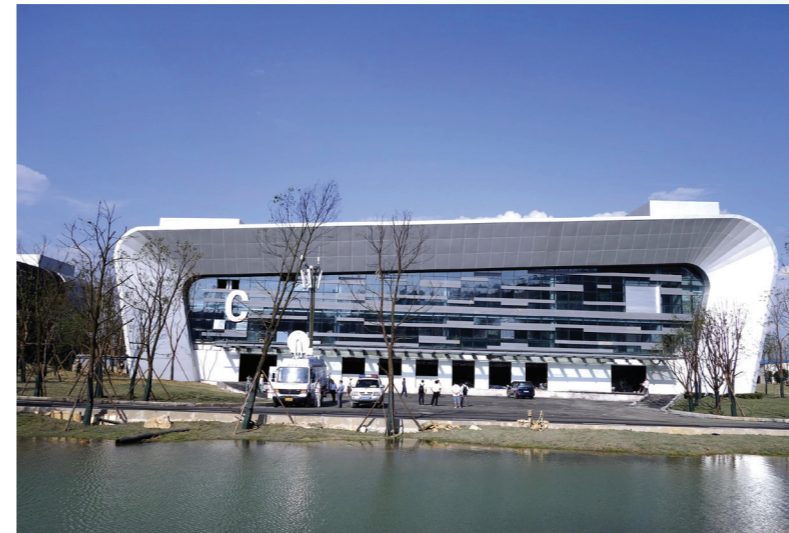
Efficient roof panel design at the Guizhou facility
