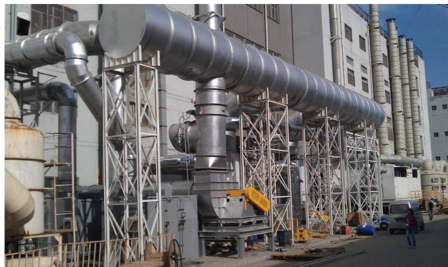
Air pollution control via the ERCO exhaust treatment system
